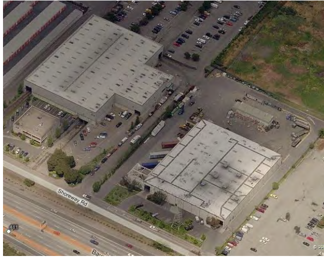
Existing Site Prior to Upgrades
