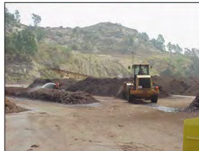
Griffith Park Composting Facility
