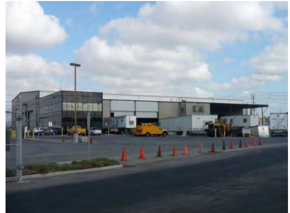
Central Los Angeles Recycling & Transfer Station
