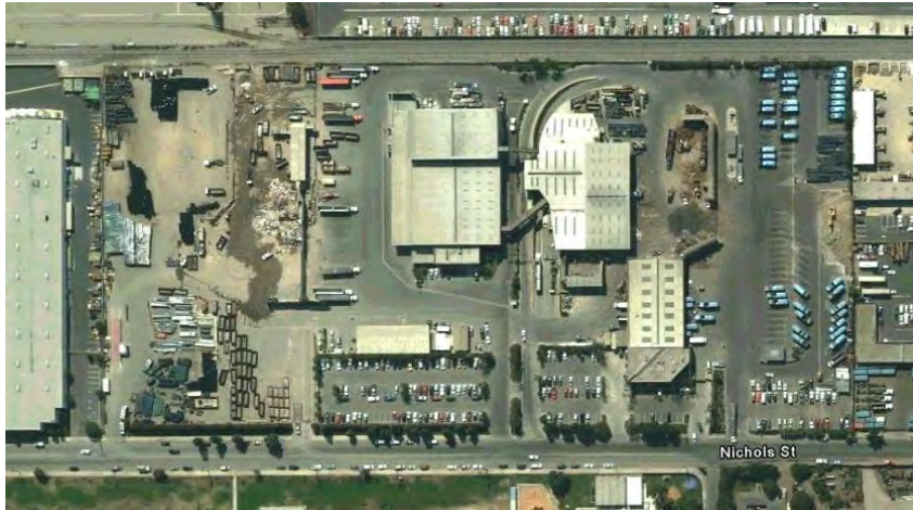
Existing Site Prior to Upgrades
